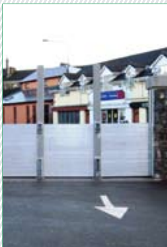
Demountable partially erected in preparation for flood.
